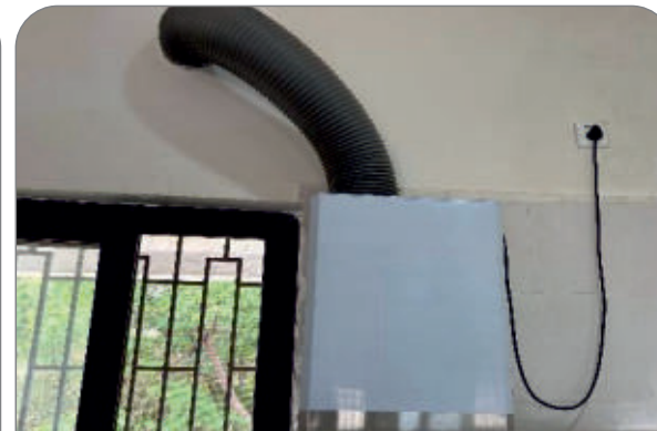
Chimney in Non-Veg Section
