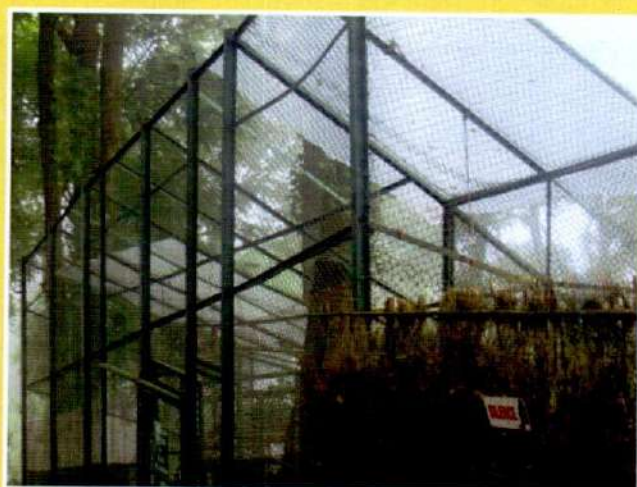
Renovation of Langur enclosure
