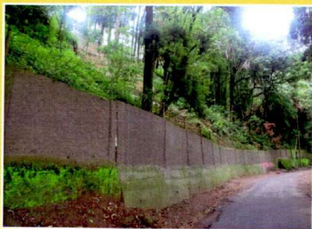
Emergent restoration of landslide
