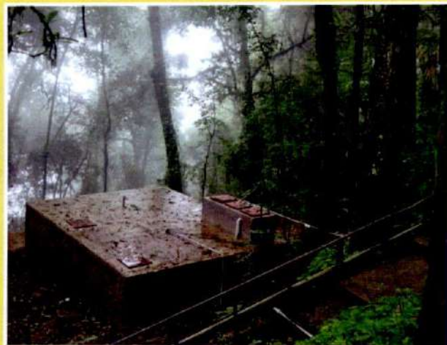
Construction of water reservoir
