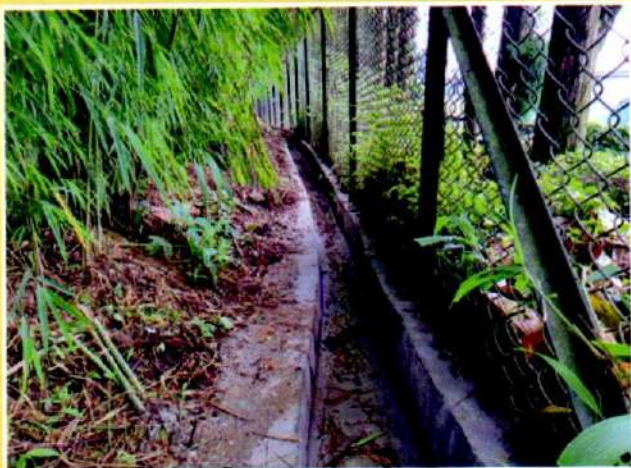
Construction and Repair of drains
