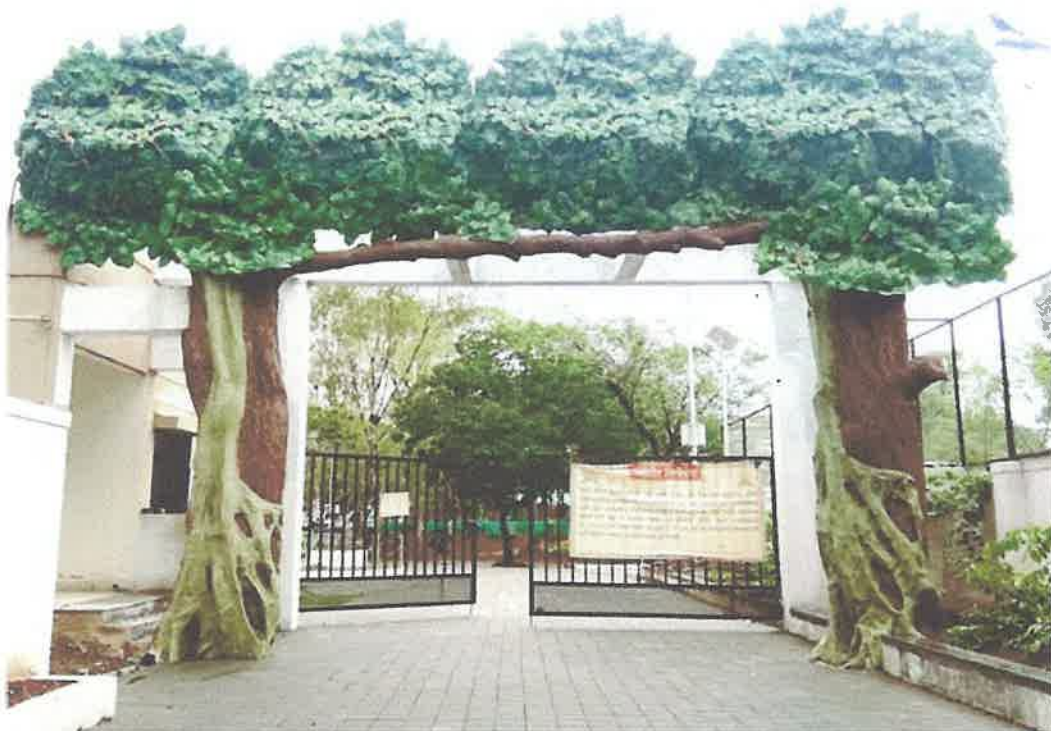
CURRENT STATUS OF ENTRANCE GATE
