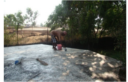
Painting lime to roof of animal house.
