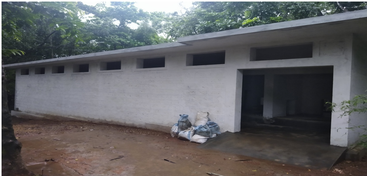
Extension of animal quarantine (under construction)
