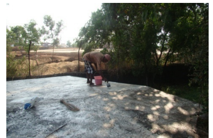
Painting lime to roof of animal house.
