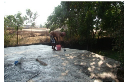
Painting lime to roof of animal house.
