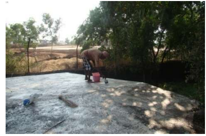
Painting lime to roof of animal house.
