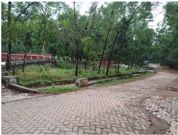
Pavement of interlock for visitor's path and service roads
