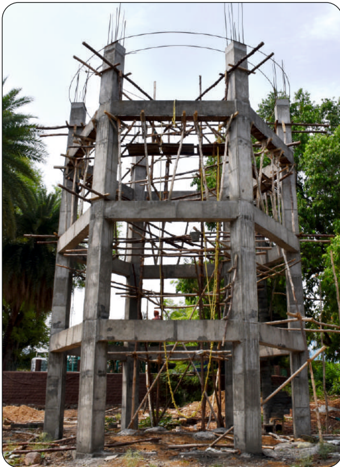
OHSR Under construction
