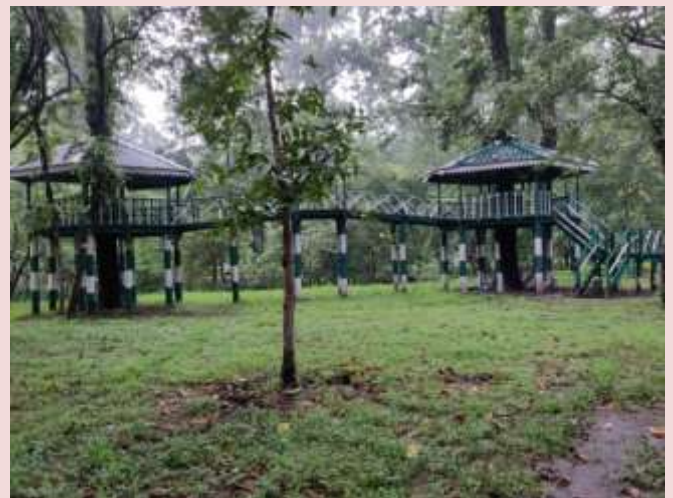
Fig: Repairing of Wooden Bridge
