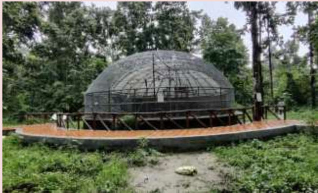
Fig: Replacement of SS Net with GI chain link at AV-3
