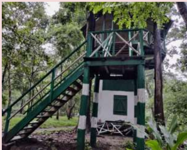
Fig: Repairing of Tree Tower
