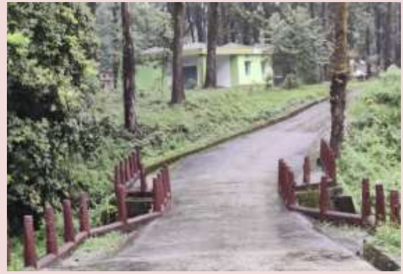
Fig: Pick up point culvert railing
