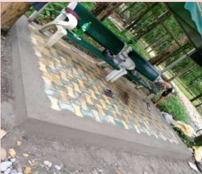
Fig: Modification at visitors seating area
