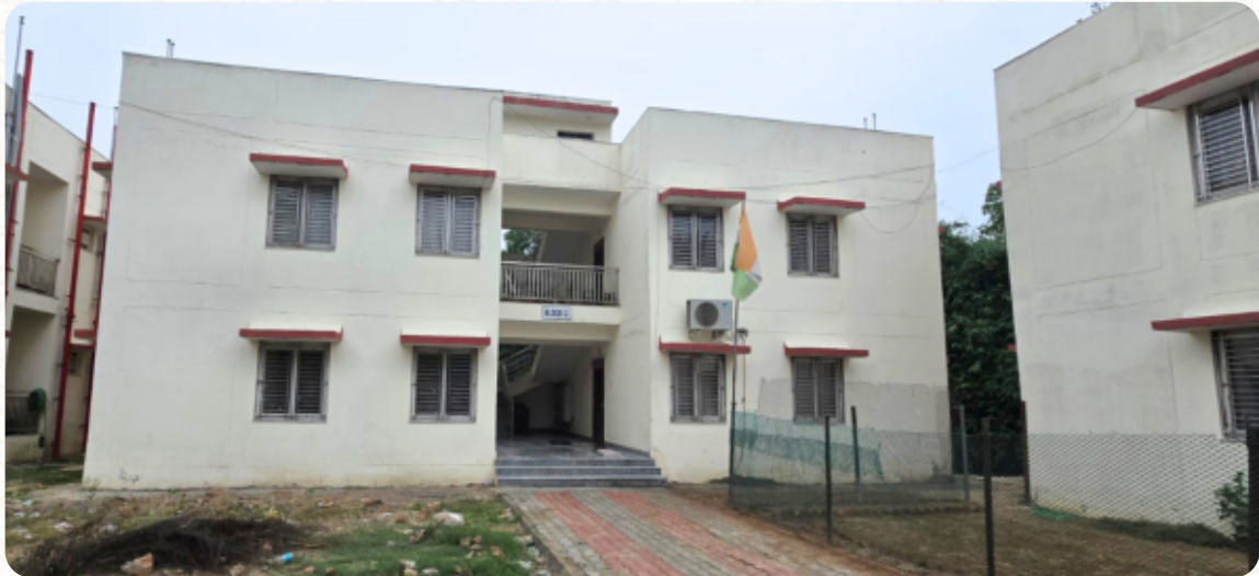
Newly Constructed quarters
