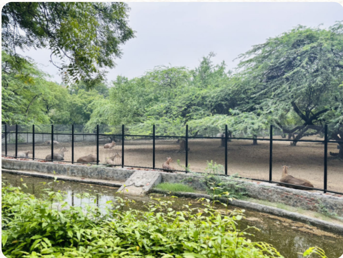
Providing and fixing chain link fencing at Deer Enclosure beat no.06
