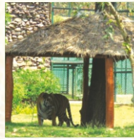
Eco friendly thatching to provide shelter from sun and rain
