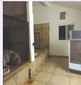
Air cooler erected at night shelters of enclosures
