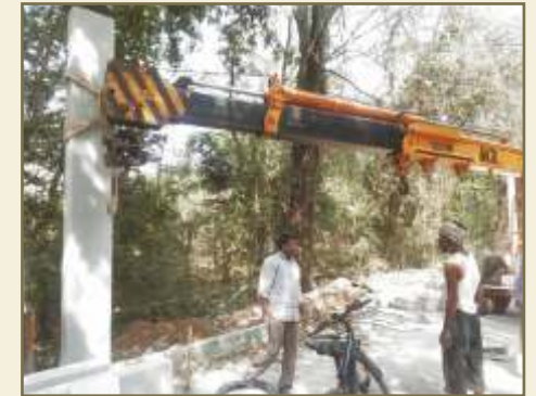
B 2. Replacement of Stone Pillars at Thandi Sadak at Zoo
