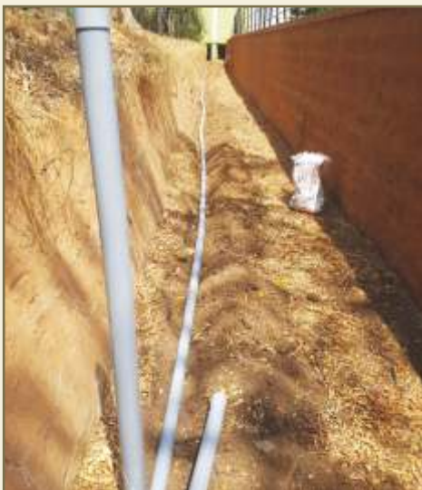
B 15. Installation of Jet Sprinkler for Giraffe Enclosure
