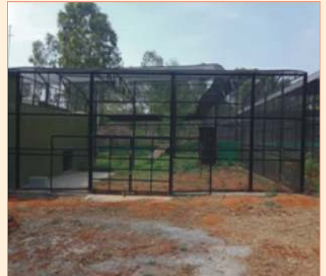
Construction of additional day kral at Rescue Centre
