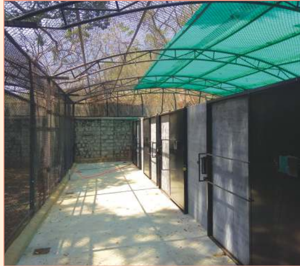
Construction of quarantine facility
