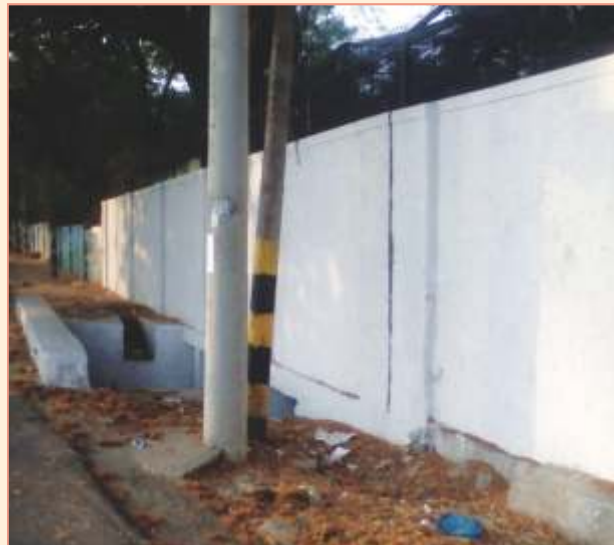
Reconstruction of weak compound wall near crocodile enclosure
