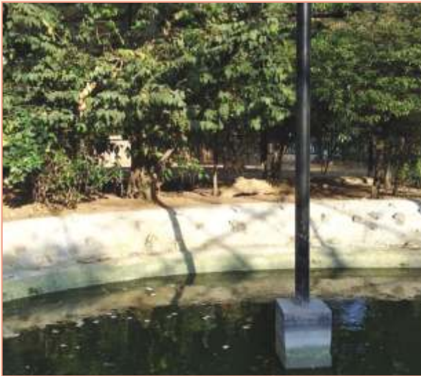
Renovation of Japan Pond
