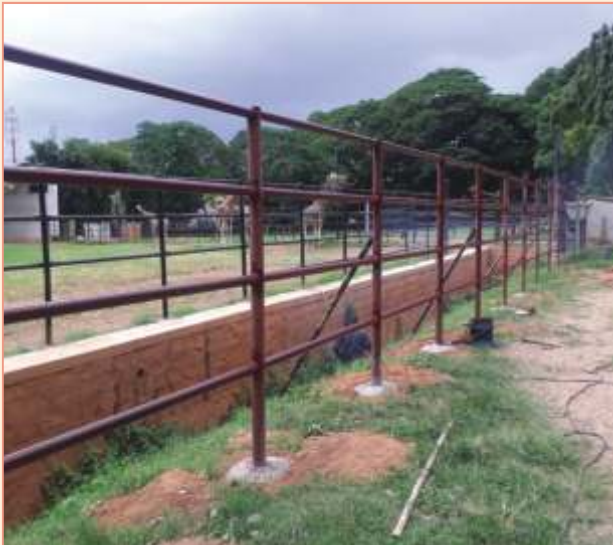
Repair & painting of railings at Giraffe enclosure
