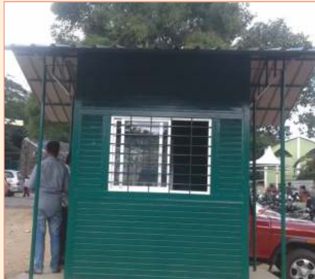
Installation of monitor room at Zoo Parking
