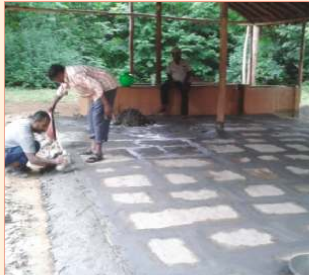
Repair of feeding platform of Zebra
