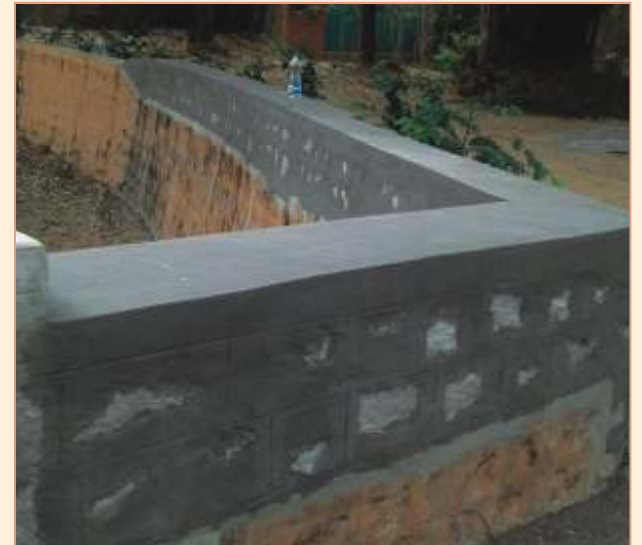
Up-gradation of moat wall of Gaur enclosure
