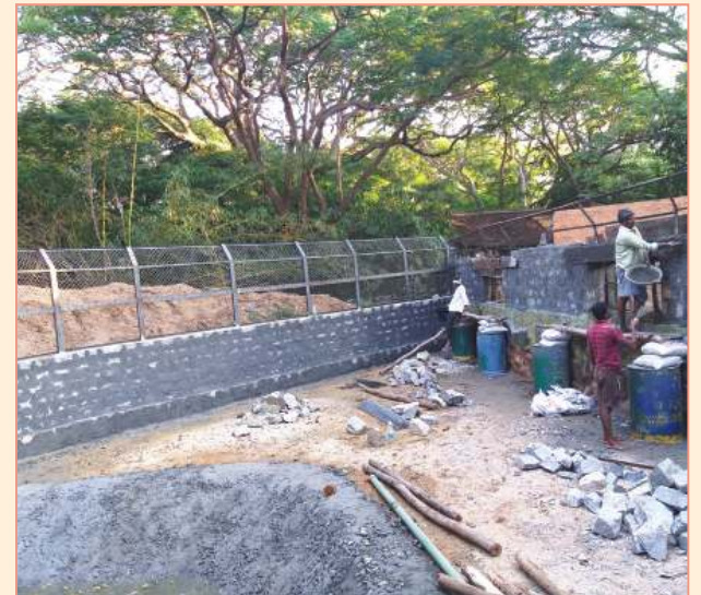
Construction of additional Hippo enclosure
