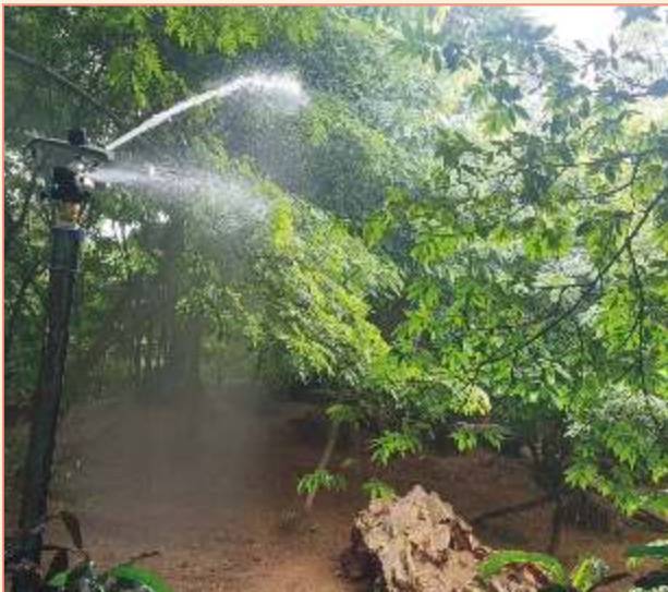
Installation of sprinklers at animal enclosures to manage heat.
