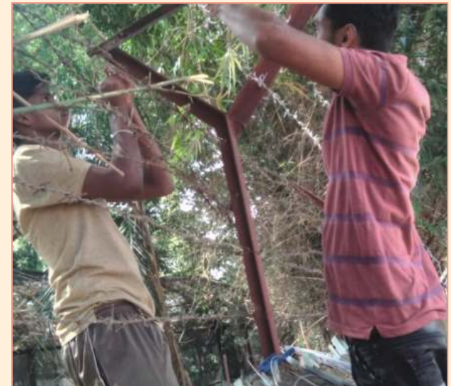
Repair of Zoo fence
