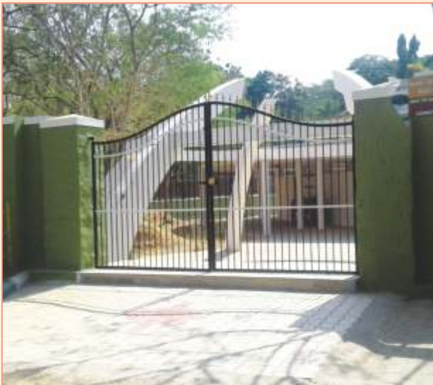
Construction of path connecting Zoo and Karanji Lake
