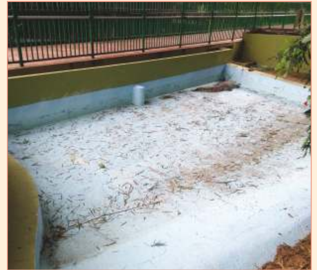
Renovation of Marsh Crocodile enclosure to avoid seepage of water
