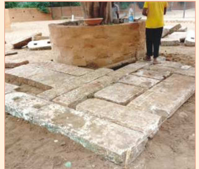
Construction of feeding platform at Spotted deer enclosure
