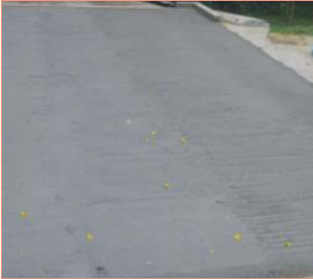
Repair of weighing machine ramp
