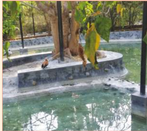
Renovation of Japan Pond
