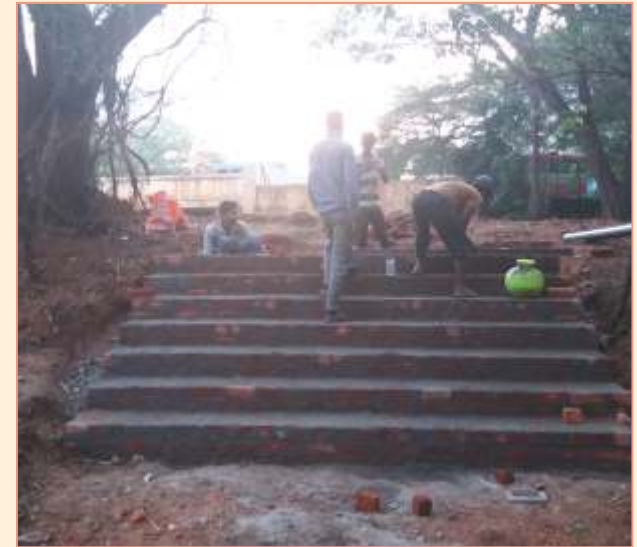
Construction of path connecting Zoo and Karanji Lake
