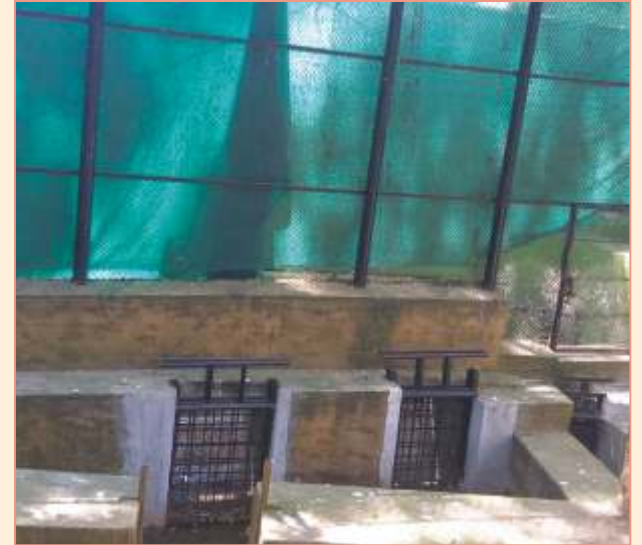
Construction of drain canal gates in open aviary enclosure
