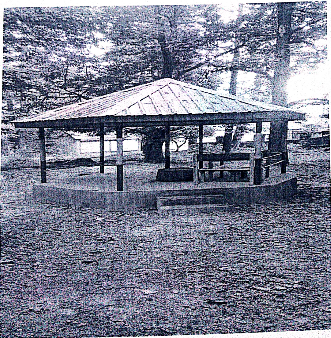
3. Construction of Rain shulter at Nehru pheasantry.
