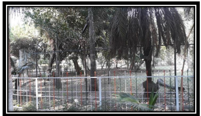
Photograph III: Showing newly constructed Emu's enclosure
