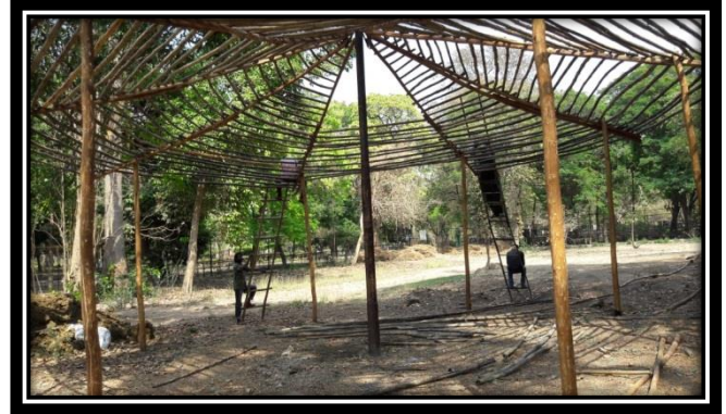
Photograph III : Showing construction of shed for Nilgai in new enclosure.
