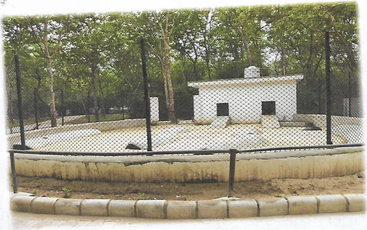
Renovation of Porcupine Enclosure
