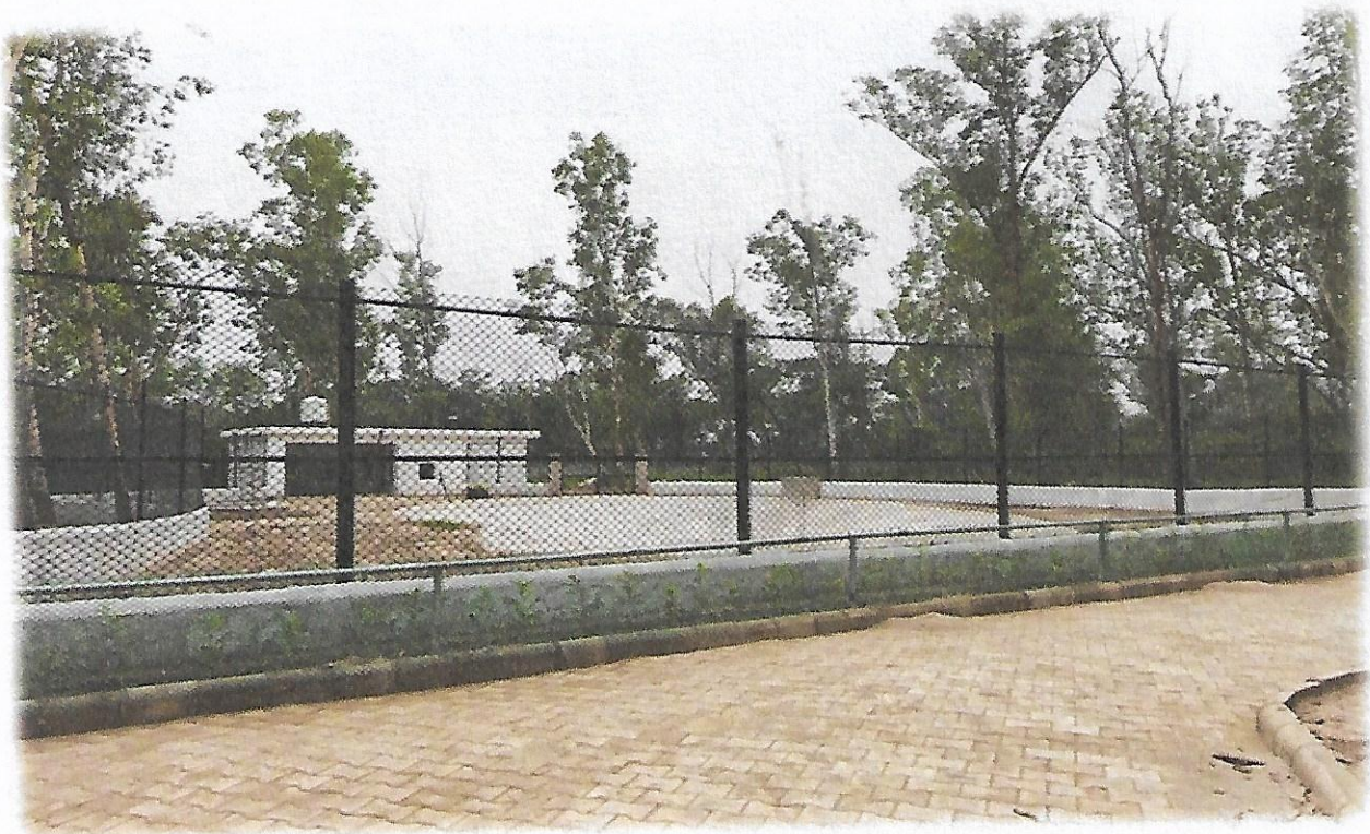
Construction of New Gharial Enclosure
