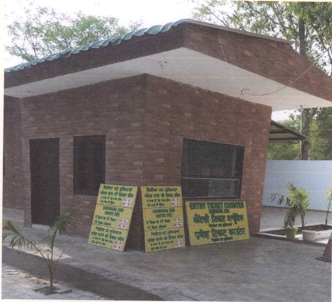
Renovated Ticket Counter
