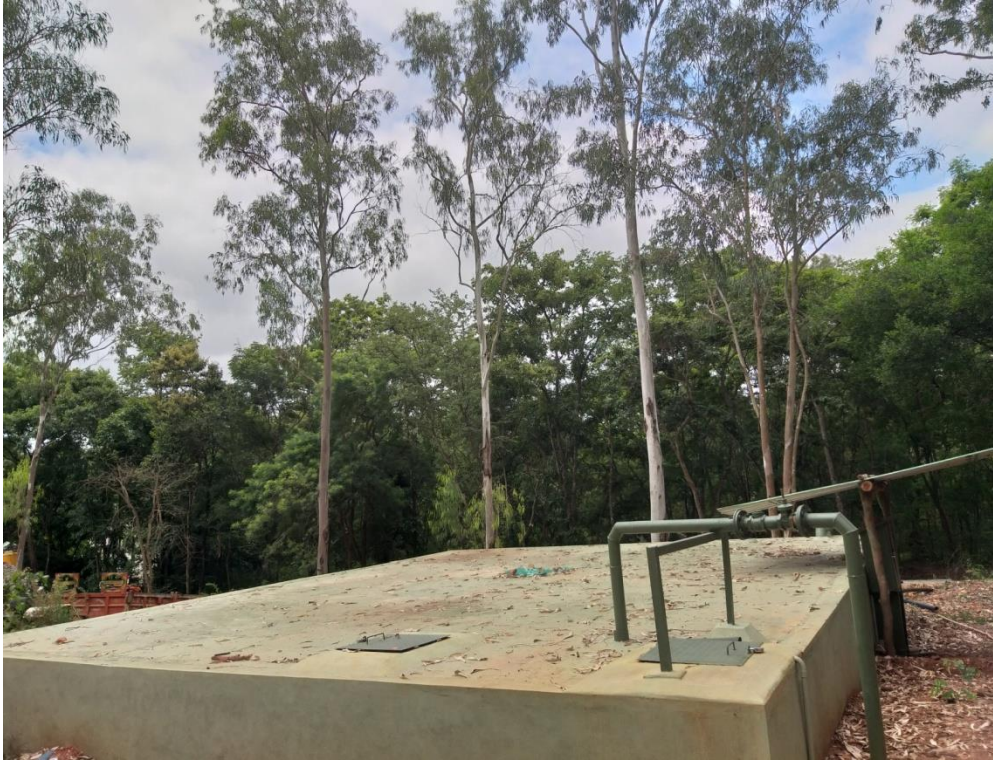
Construction of 2.00 lakh capacity GLSR at Tiger & Lion Safari
