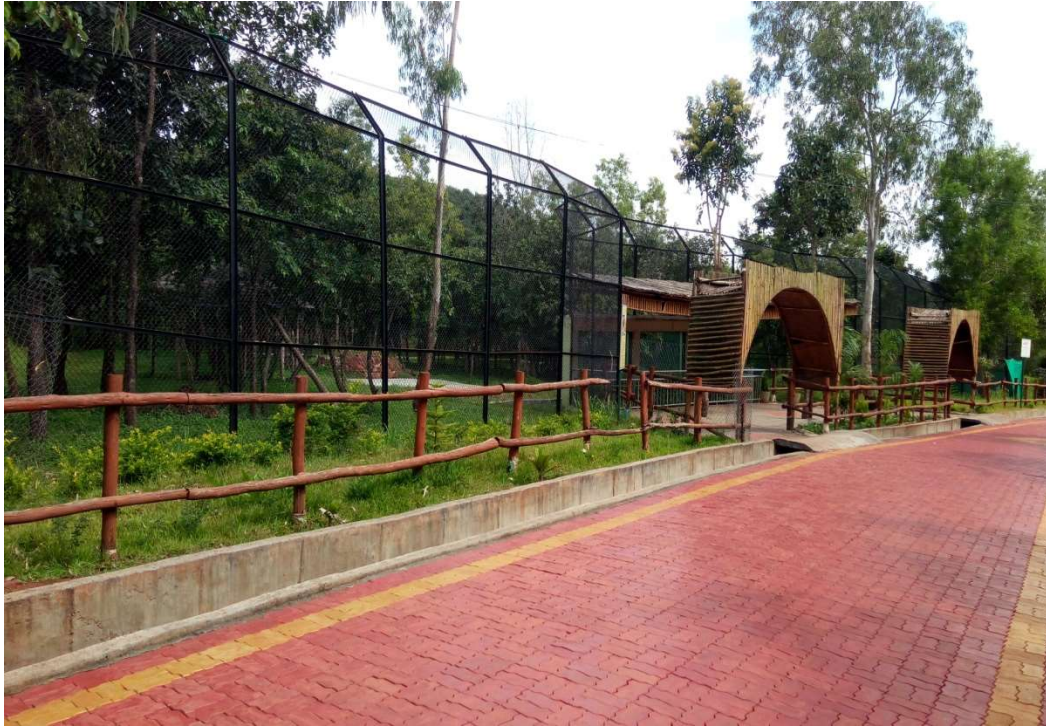
Shade Structure Infront of Lion Enclosure
