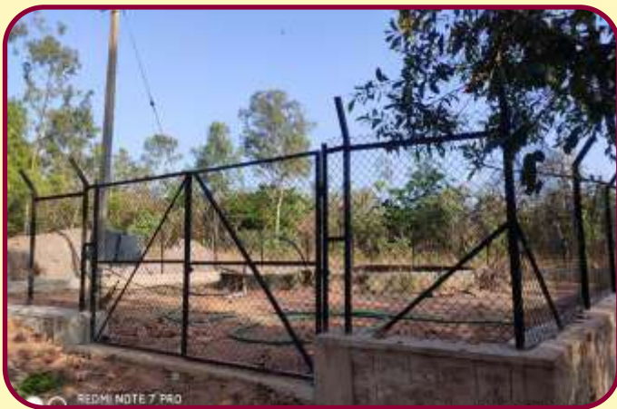
Fencing for open Well
