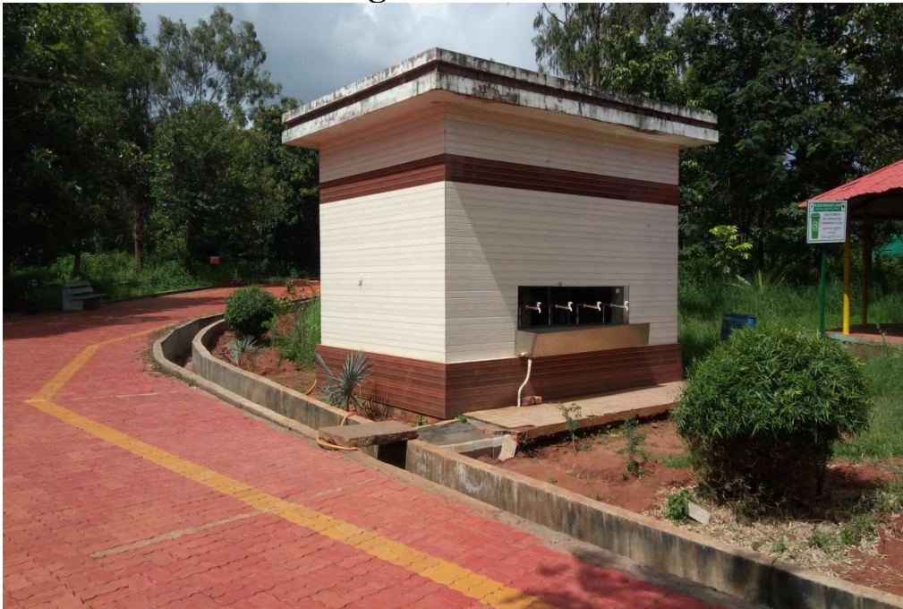
Drinking Water R.O Plant
