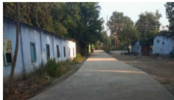
Newly constructed service road.
