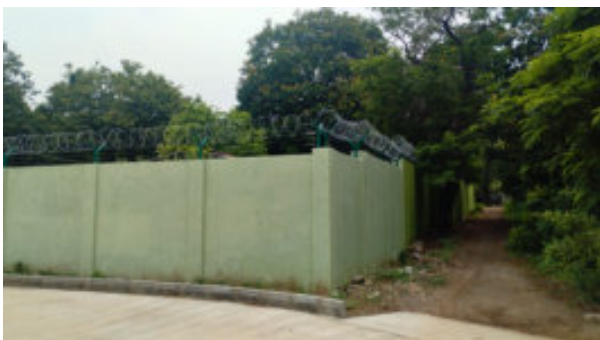
Newly constructed perimeter wall.
