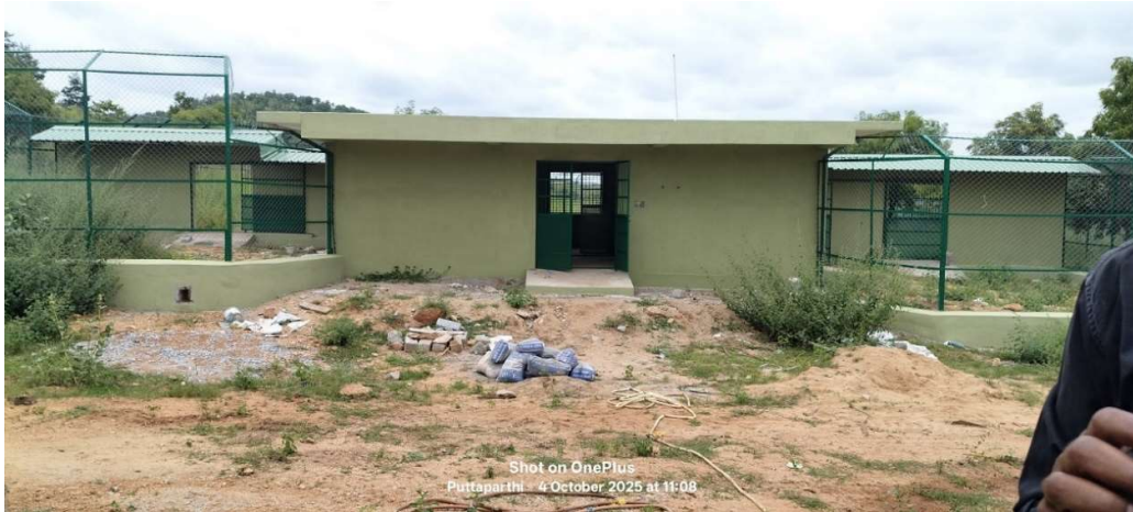
Deer enclosure 2 completed
