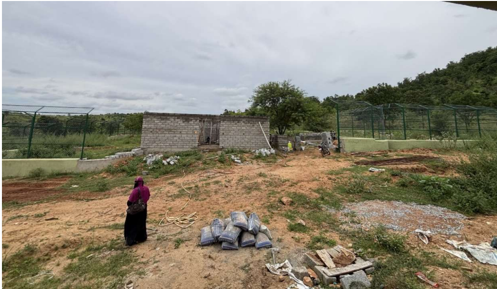
Deer enclosure 3 under construction
