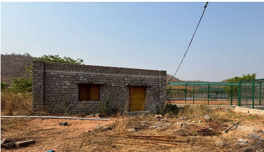
Kitchen & store room inside view
