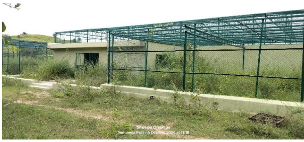
Monkey enclosure1 completed
