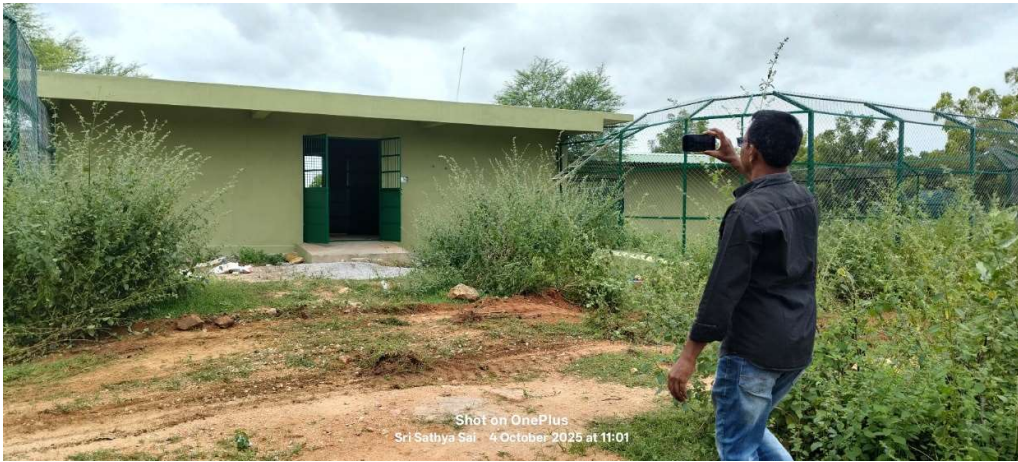
Deer enclosure 1 completed
