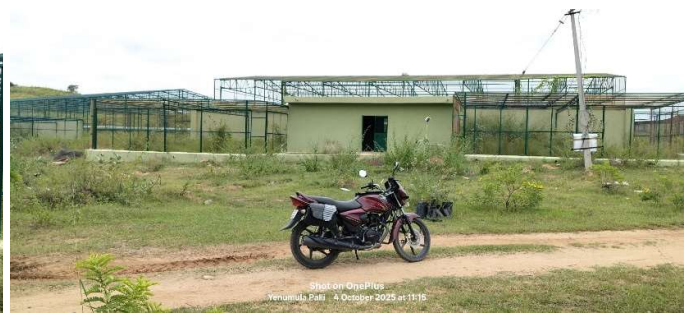
Monkey enclosure2 completed
