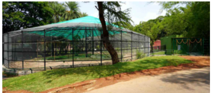
The old wet moats of primates were converted into dry enclosures, providing increased space to accommodate the troop and ensuring better movement within the habitat.
