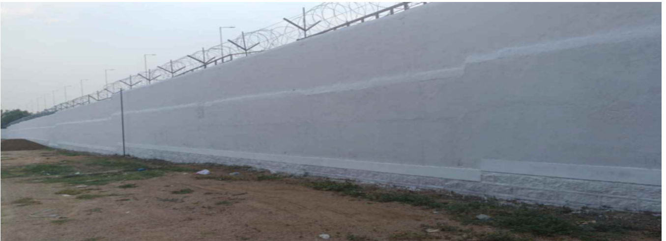
Electric Fencing was installed during this year
