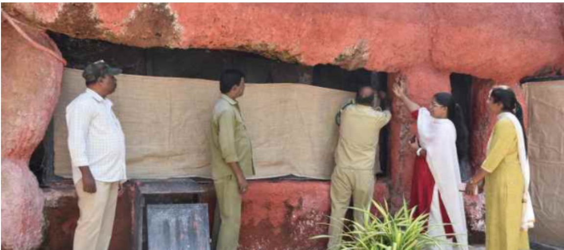
As a part of winter arrangements, the windows and doors are covered gunny rolls inorder to prevent cool breeze
