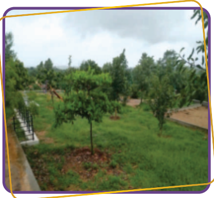
New compound wall for childrens park
