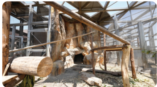
The Baboon Enclosure has been enhanced with new ferro-work, additional shade structures, and enrichment elements, designed to improve comfort, behavioral stimulation, and overall welfare for the residents.
