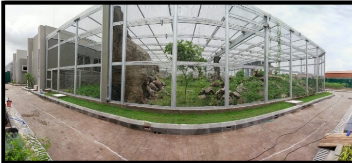
Side profile of an enclosure at the extension of Satellite Rescue Centre for leopards
