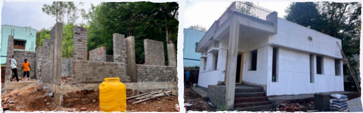
Curator/RFO Quarters Construction
