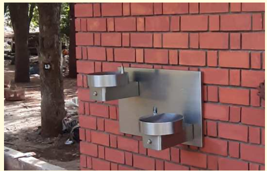
RO Drinking Water Plant
