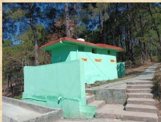
Image 11 Painting and repair work of toilet facilities
