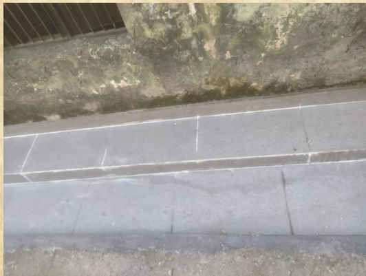
Image 7 Repair of drain in Leopard indoor holding area
