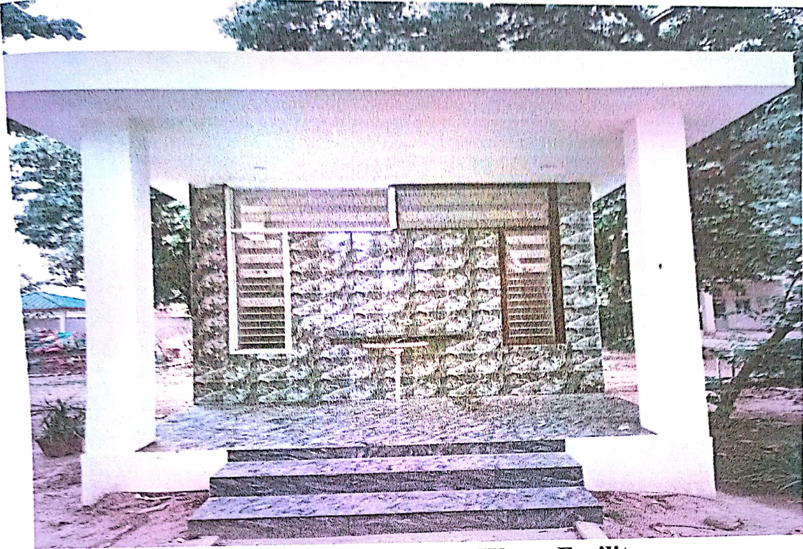
Creation of One Drinking Water Facility
