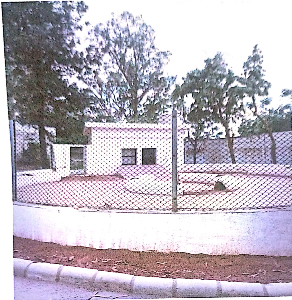
Renovation of Porcupine Enclosure
