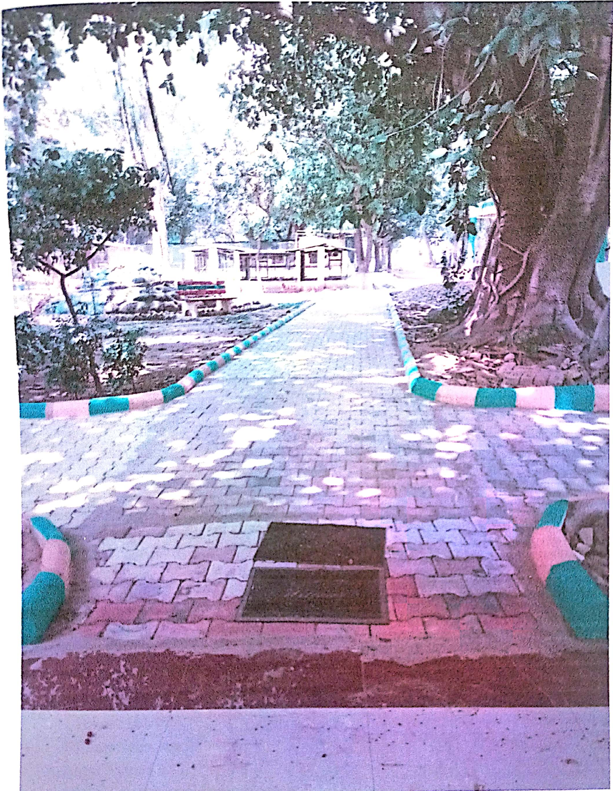
Repair of Visitor path through interlock tiles
