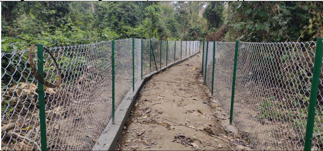
Figure c: The open outdoor enclosure partitioned into two by erecting a double row chain-link mesh barrier that permits keepers to walk in between.
