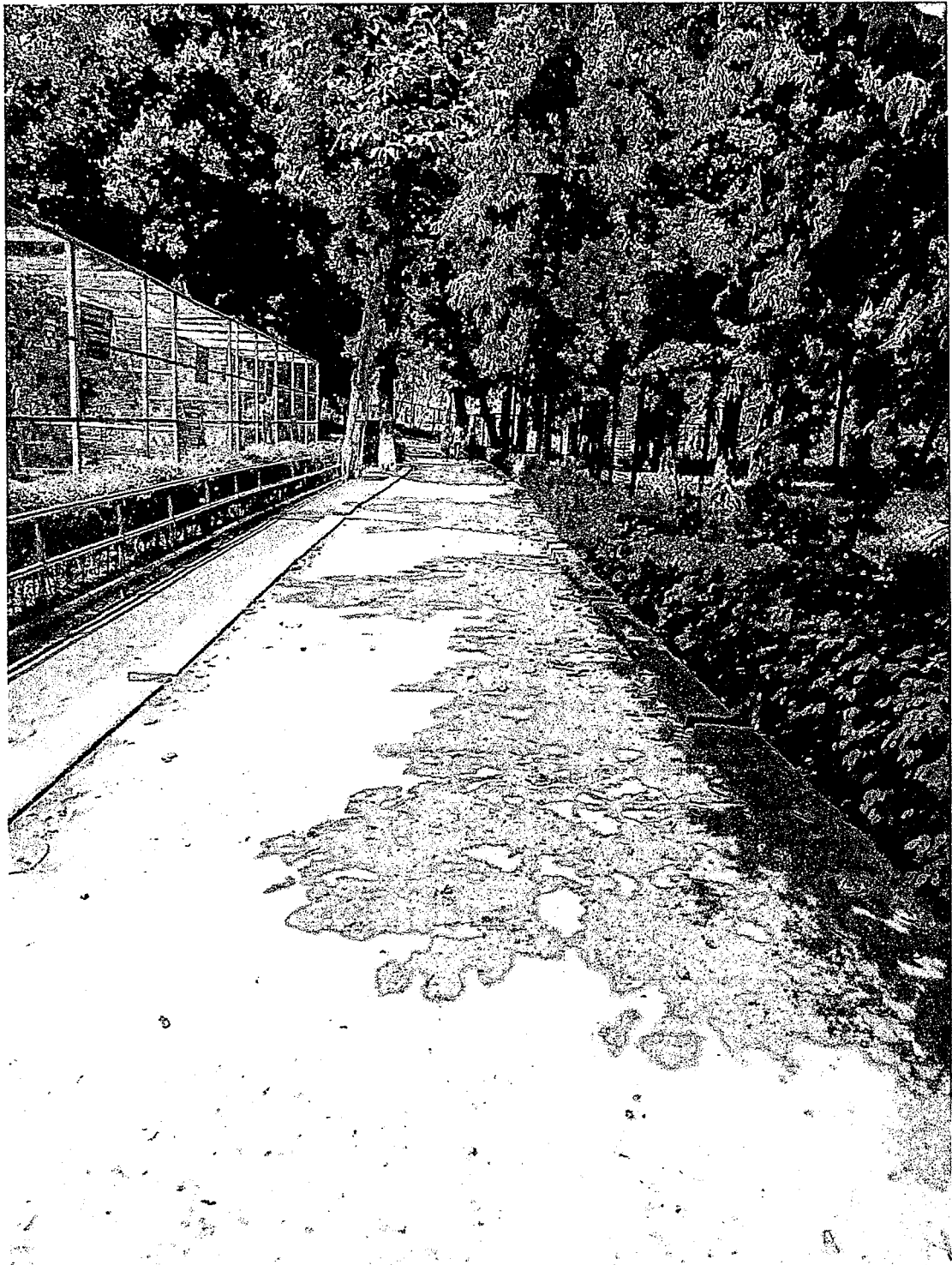
Construction of Concrete Road for Visitor's Path at Bardhaman Zoological Park
