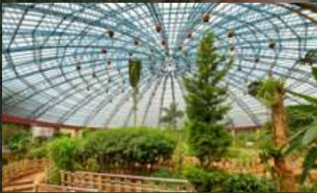
Earthen Pots hung for Acoustic Control to avoid eco sound
