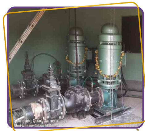
Construction of Jack well
