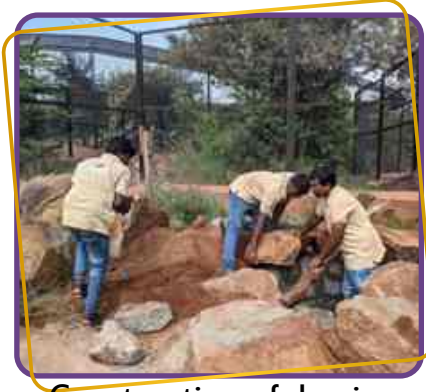
Construction of den in hyna enclosure
