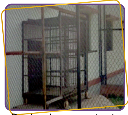
Day kraal construction in hospital area
