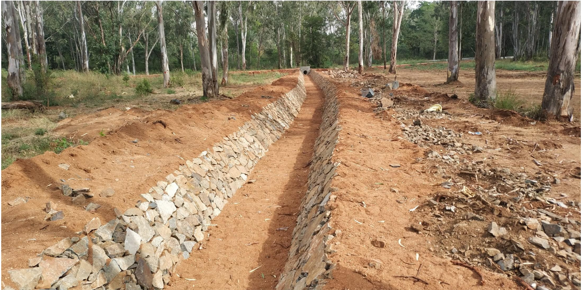
Feeder channel between two pond
