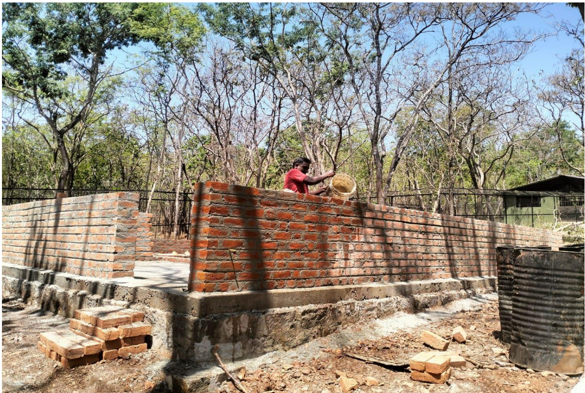
Construction of Toilet Block (next to nilgai enclosure) during 2022-23
