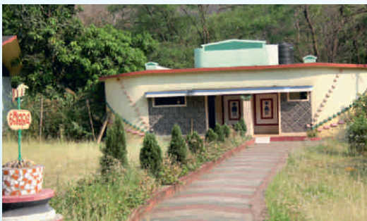
Public Convenience Complex
