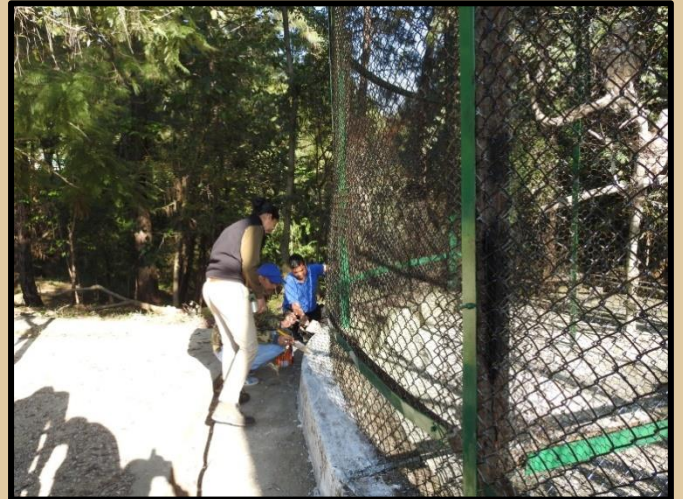
Picture 8: Outer fence maintenance near Birds of Prey enclosure.
