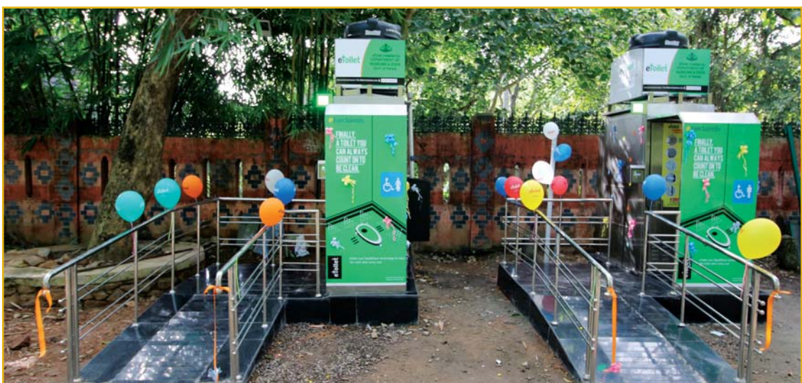
Access ramp for PwDs toilet
