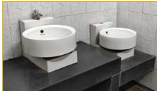
Wash basins provided at two levels for PwDs and children
