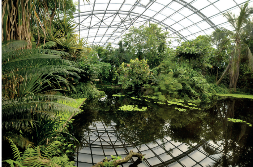
Figure 1: The Masoala Rainforest exhibit is spanned by a 30 meter tall and 90 meter wide, highly translucent ETFE roof construction. Credits: Zoo Zurich, Martin Bauert.
