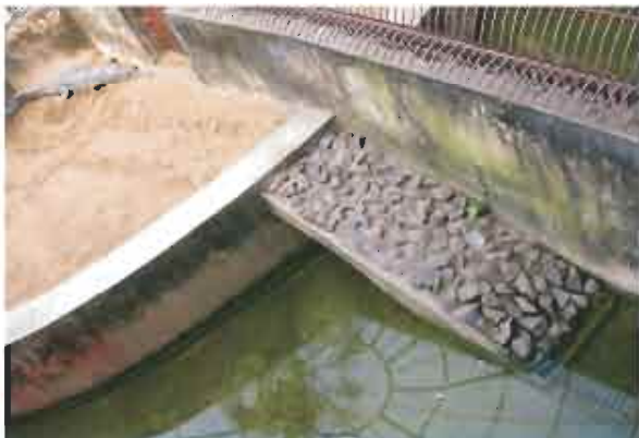
Sharp edged stones may cause injuries to animals and hence should be avoided.
