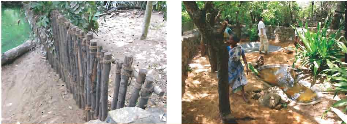
Erected temporary barrier (left) to facilitate cleaning (right).
