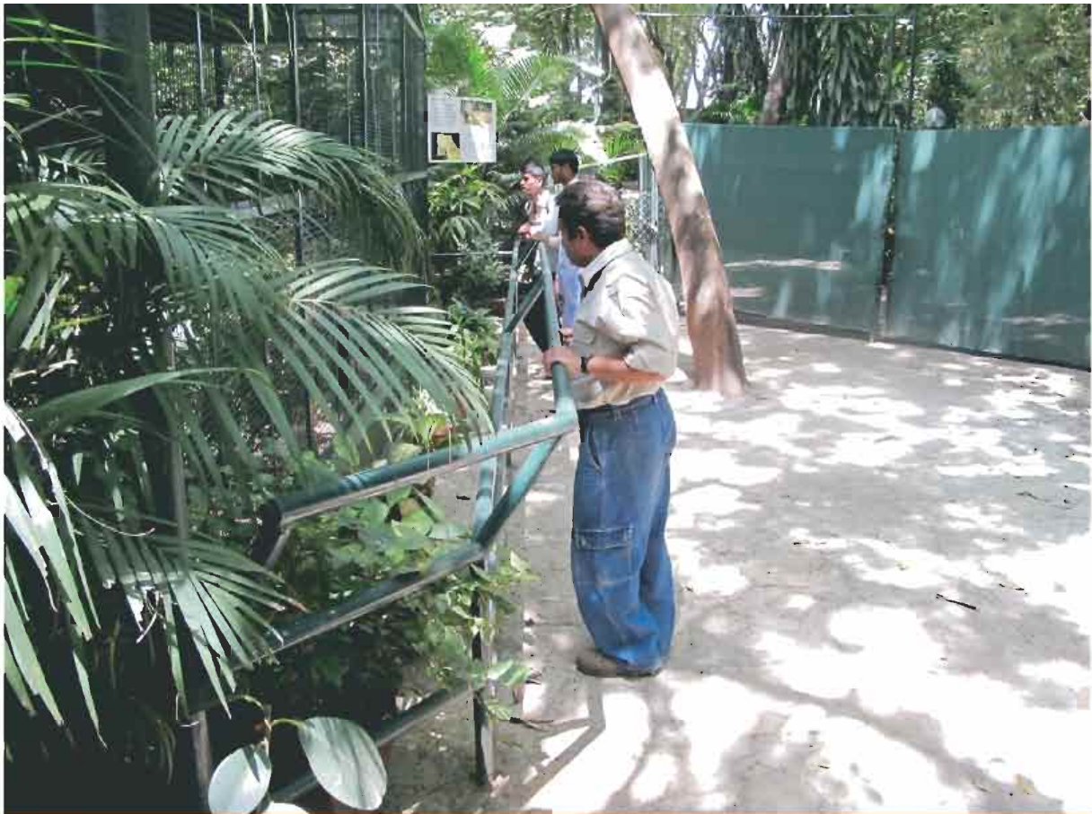
The above railing design provides adequate distance between the cage and the visitors.
