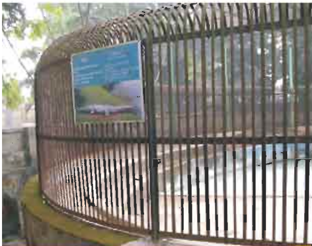
The heavy metal bars give the enclosure the look of a jail barricade which should be avoided.
