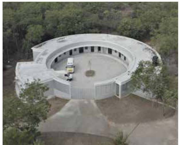
► Aerial View of Commissary Building
