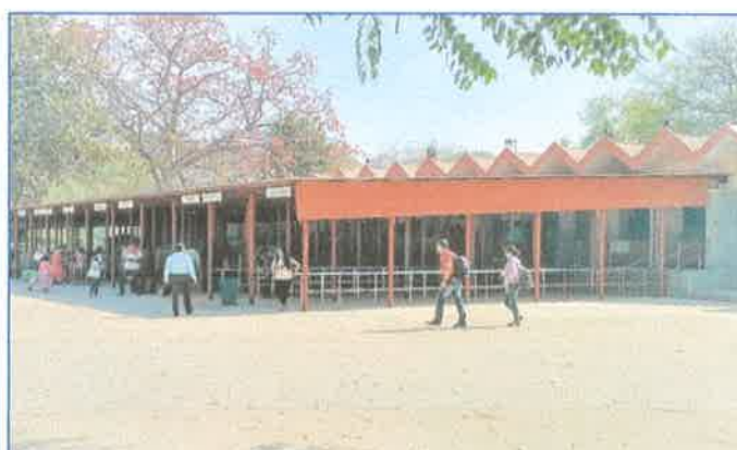
Visitor Shade at Ticket Counter
